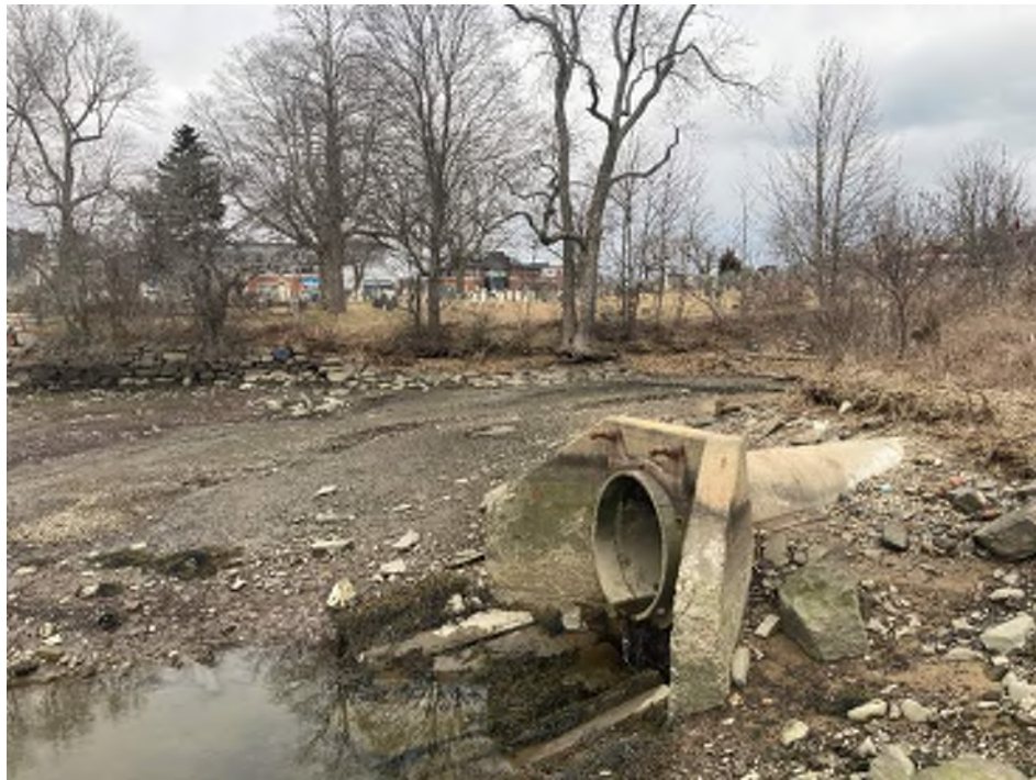
Photo 12 – Existing outfall headwall with mitigation area in background looking east at approximate low tide. Taken 3/20/24
