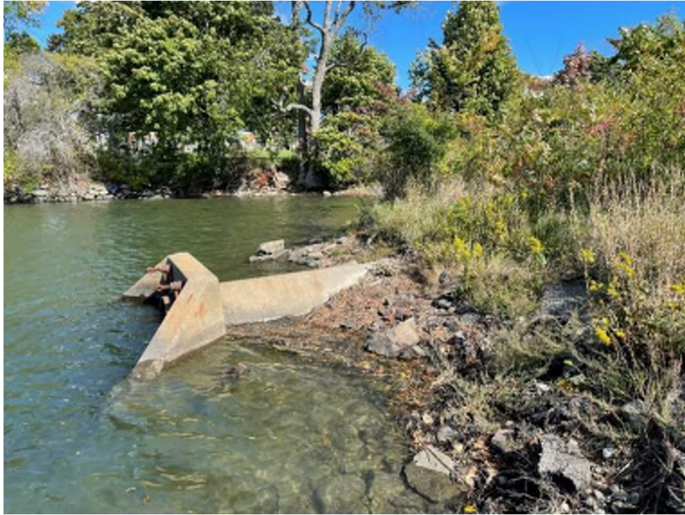
Photo 3 – Existing outfall headwall, exposed 48” RCP pipe, and tidal embankment looking east at approximate high tide. Taken 9/28/22
