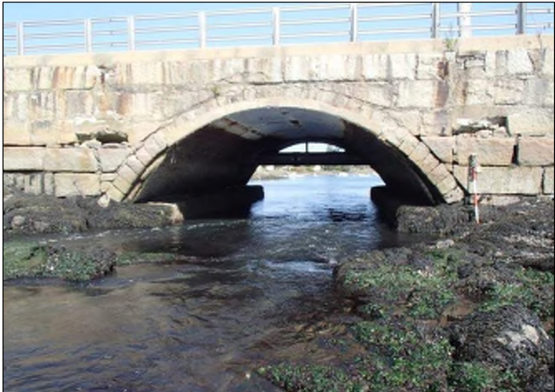
Figure 3 – View north at the existing bridge inlet (09-23-20)
