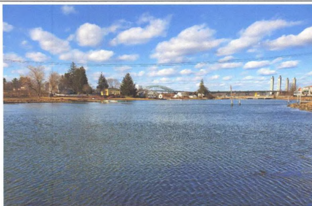
FIGURE 4 North Mill Pond, Seaward Side, View North from East Side of Culvert in Maplewood Road, Mid-Incoming Tide (2/28/2020)
