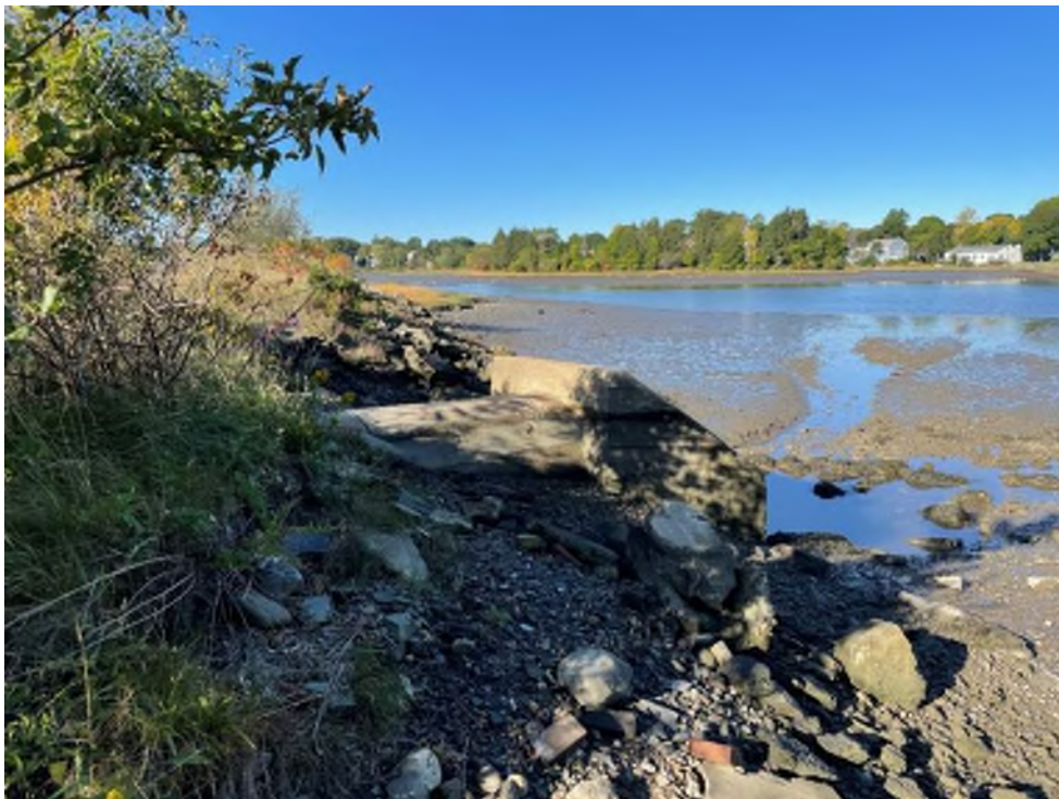
Photo 4 – Existing outfall headwall, exposed 48” RCP pipe, and tidal embankment looking west at approximate low tide. Taken 9/29/22
