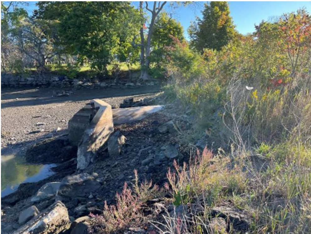
Photo 6 – Existing outfall headwall, exposed 48” RCP pipe, and tidal embankment looking east at approximate low tide. Taken 9/29/22
