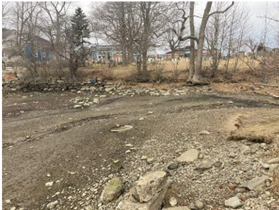
Photo 10 – Mitigation area looking east at approximate low tide. Note undercut embankment below cemetery. Marsh restoration will provide revetement. Trees and vegetation on embankment to remain, tree canopy to be trimmed up approximately 20' from ground surface. Taken 3/20/24
