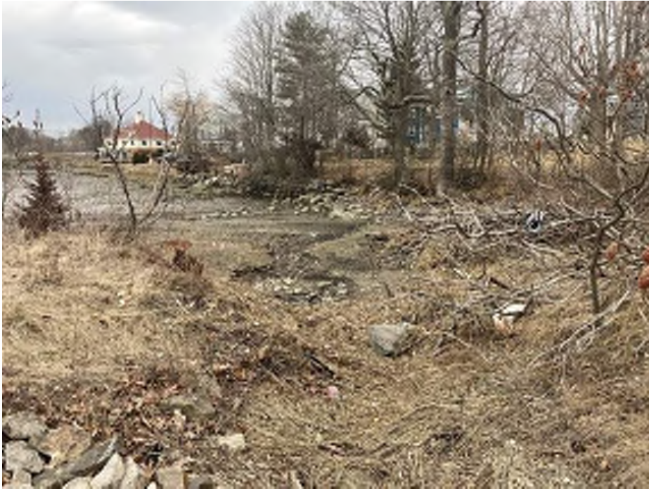
Photo 15 – Existing drainage swale outlet (to be eliminated) and erosion in mitigation area looking north at approximate low tide. Taken 3/20/24
