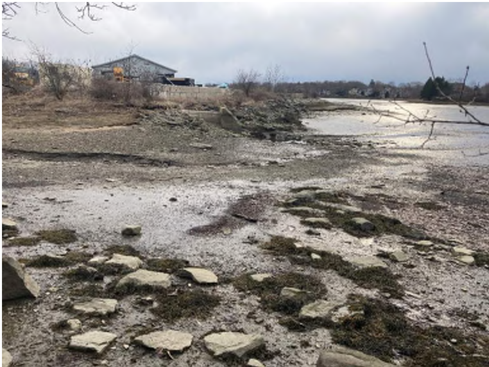
Photo 8 – Mitigation area, looking southeast at approximate low tide. Note existing large rocks to be stockpiled for use on stabilized slope and ice breakers. Taken 3/20/24
