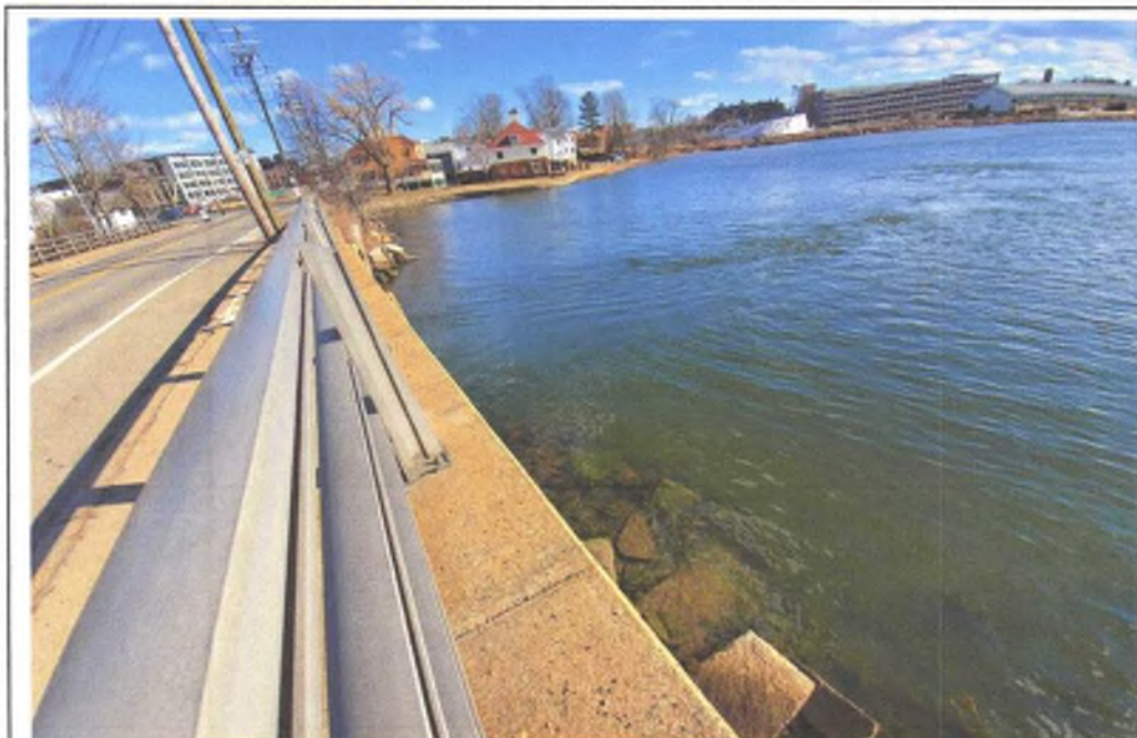
FIGURE 3 North Mill Pond, Landward Side, View Southeast from West Side of Culvert in Maplewood Road, Mid-Incoming Tide (2/28/2020)
